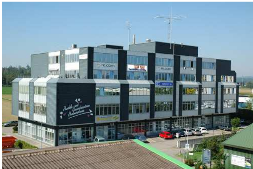
SNT Sensortechnik AG in 2nd floor of commercial center Hammerstrasse, Bülach
